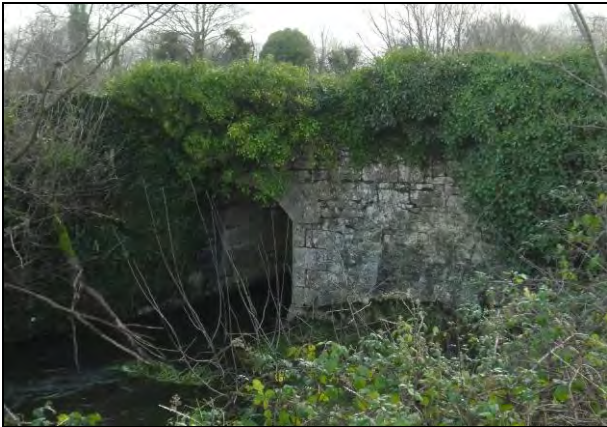
Image 14.43 Aggard Bridge (RPS 302), facing south-east
