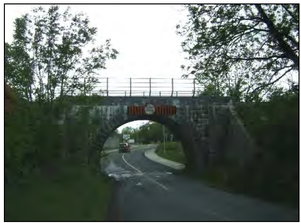
Image 14.32 Aggard Railway Bridge (NIAH 30336009), facing west
