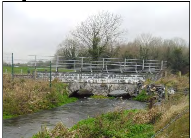
Image 14.48 Stone rail bridge in Ballynamannin townland, facing NNW
