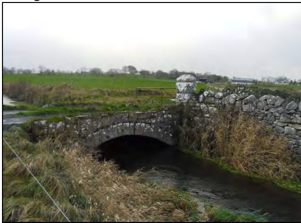
Image 14.47 Stone road bridge in Aggard Demesne, facing SSW
