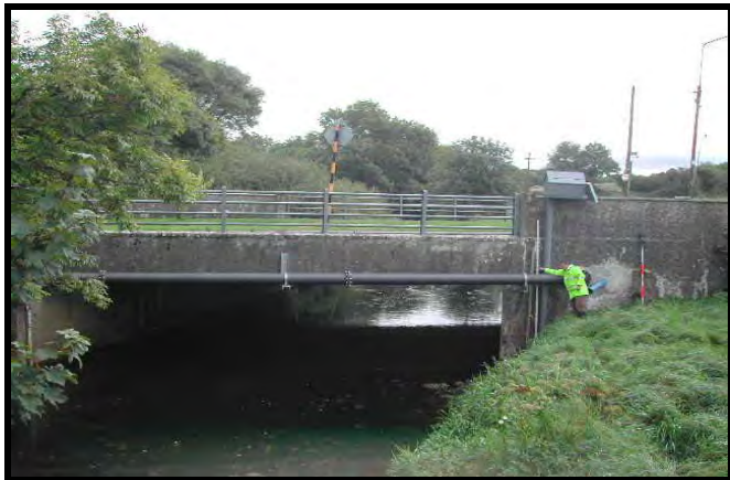
Image 17.4 R446 Bridge at Craughwell Village (formerly N6)
