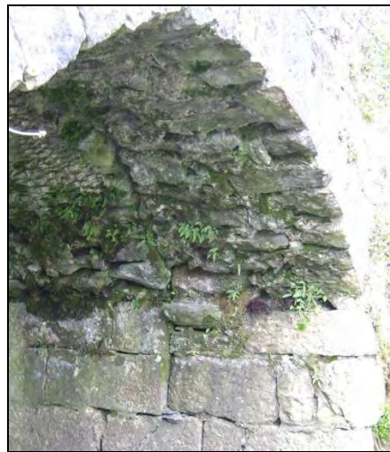
Image 14.30 Phases of construction evident at Craughwell Bridge
