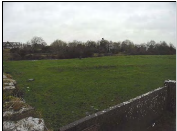
Image 14.8 Embankments to the east of Dunkellin Bridge, facing north-east
