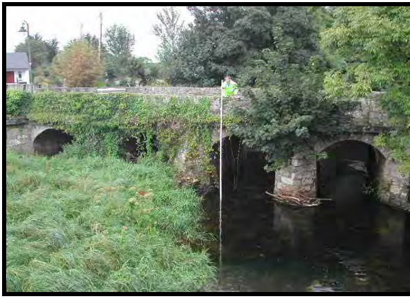
Image 17.5 Masonry Arch Pedestrian Bridge at Craughwell
