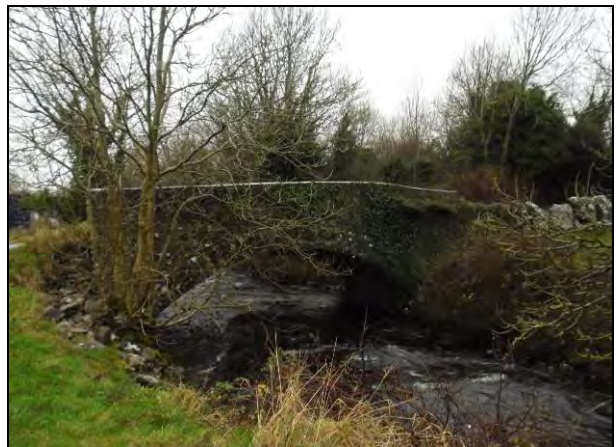
Image 14.36 Killeely Beg Bridge, facing north-west
