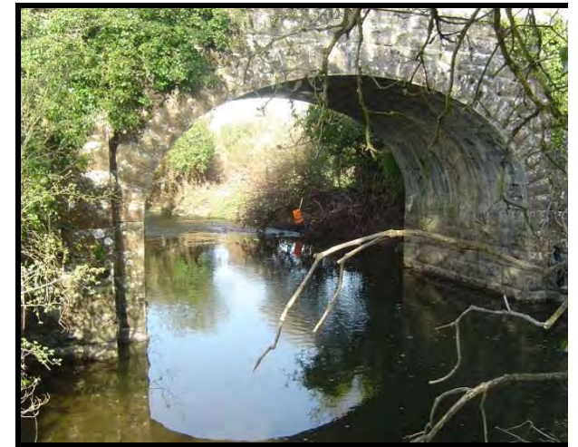
Image 17.6 Railway Bridge in Craughwell
