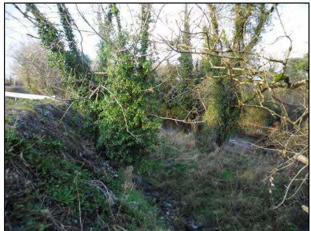
Image 14.4 Southern bank of the river, south of recent development, facing north-west
