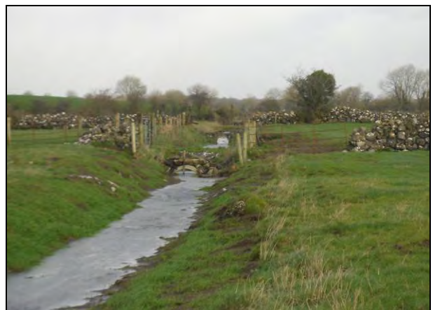
Image 14.50 Culverts AG2-4, facing south-west
