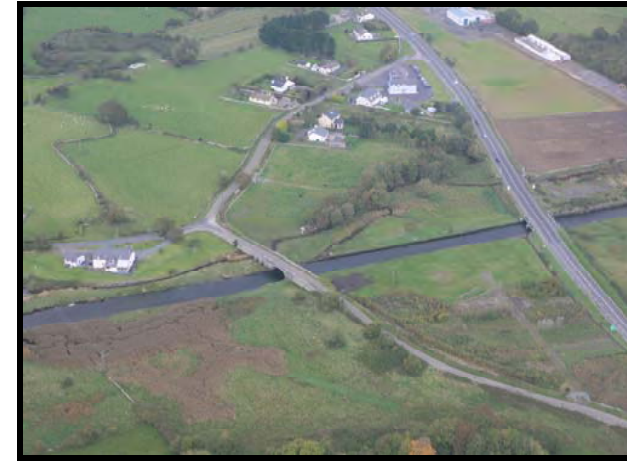
Image 17.9 N18 Kilcolgan Bridge
