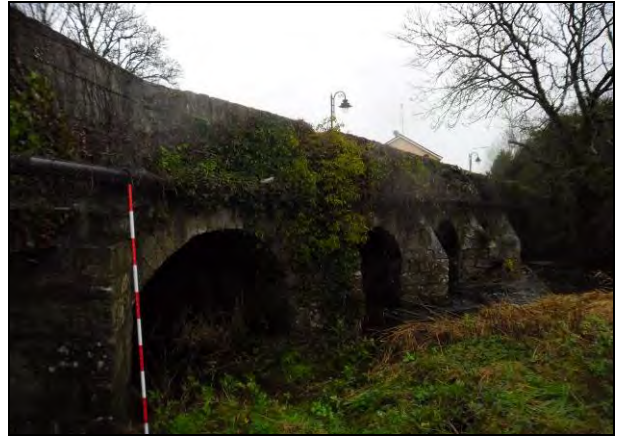
Image 14.28: Old Craughwell Bridge (NIAH 30336010), facing NNW
