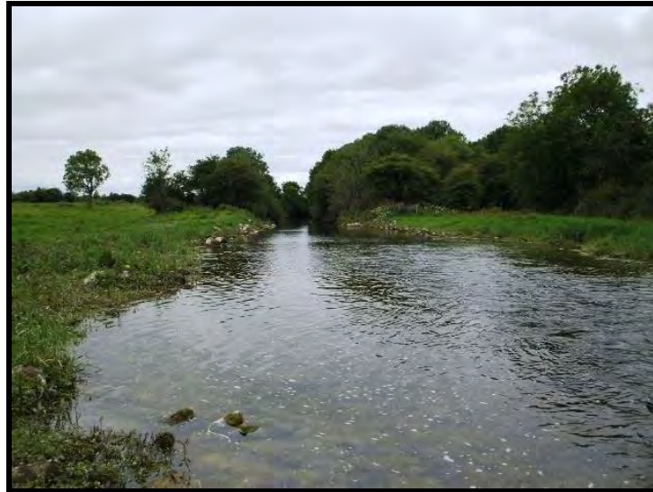
Image 15.6 View Available Below Dunkellin Bridge
