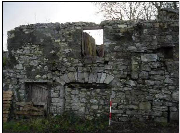
Image 14.40 Building attached to the western façade of the mill structure, facing south
