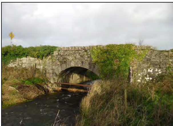
Image 14.49 Stone road bridge in Ballynamannin townland, facing NNW
